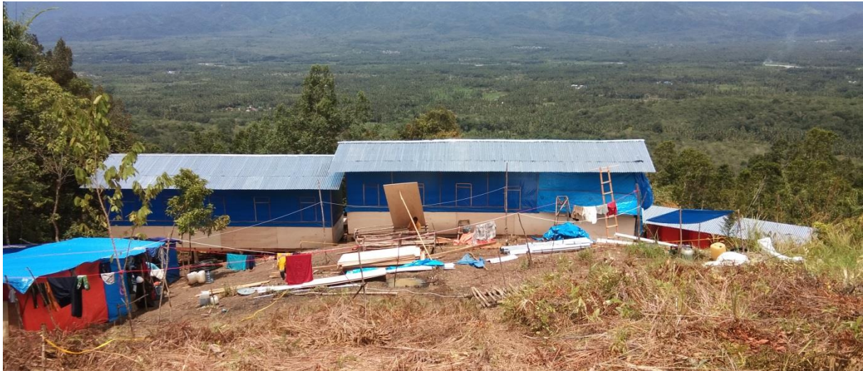
Figure 4: Tor Sigompul Camp Construction over-looking the Panyabungan Graben
