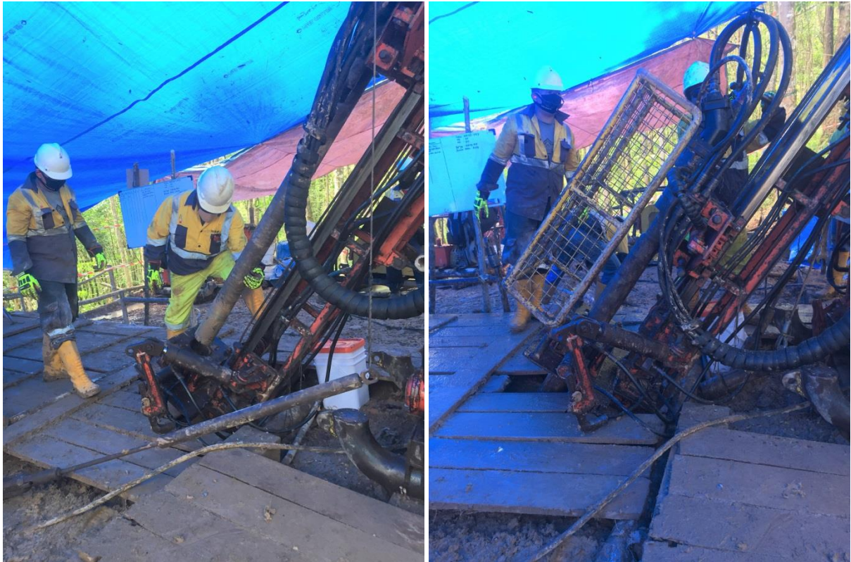
Figure 7: Hutabargot Julu – Spudding of the first drill hole HUTDD057
