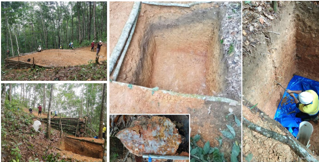
Figure 5: Hutabargot Julu – Drill pad preparations & altered volcanic bedrock in drill sumps
