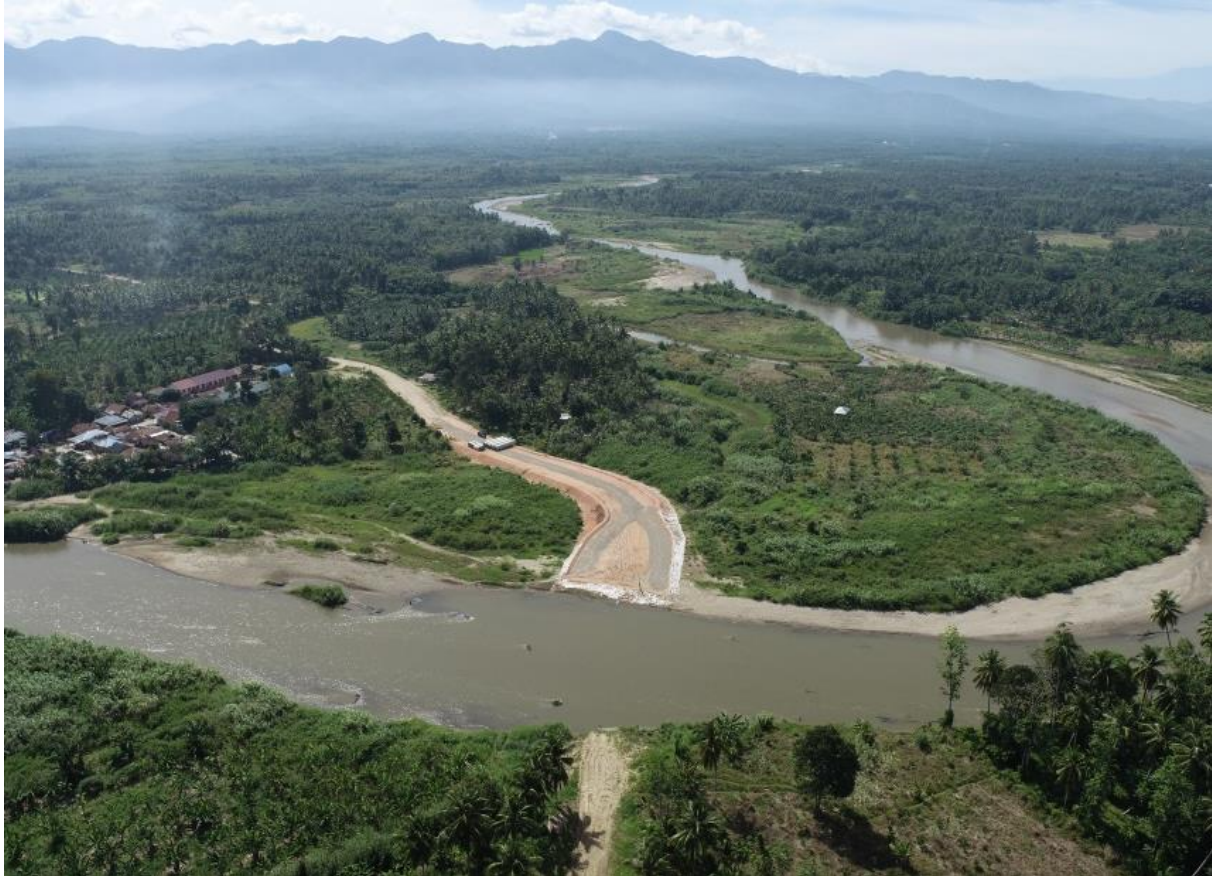
Figure 14: Current condition of Government Access Road following upgrades showing planned location of Batang Gadis Bridge
