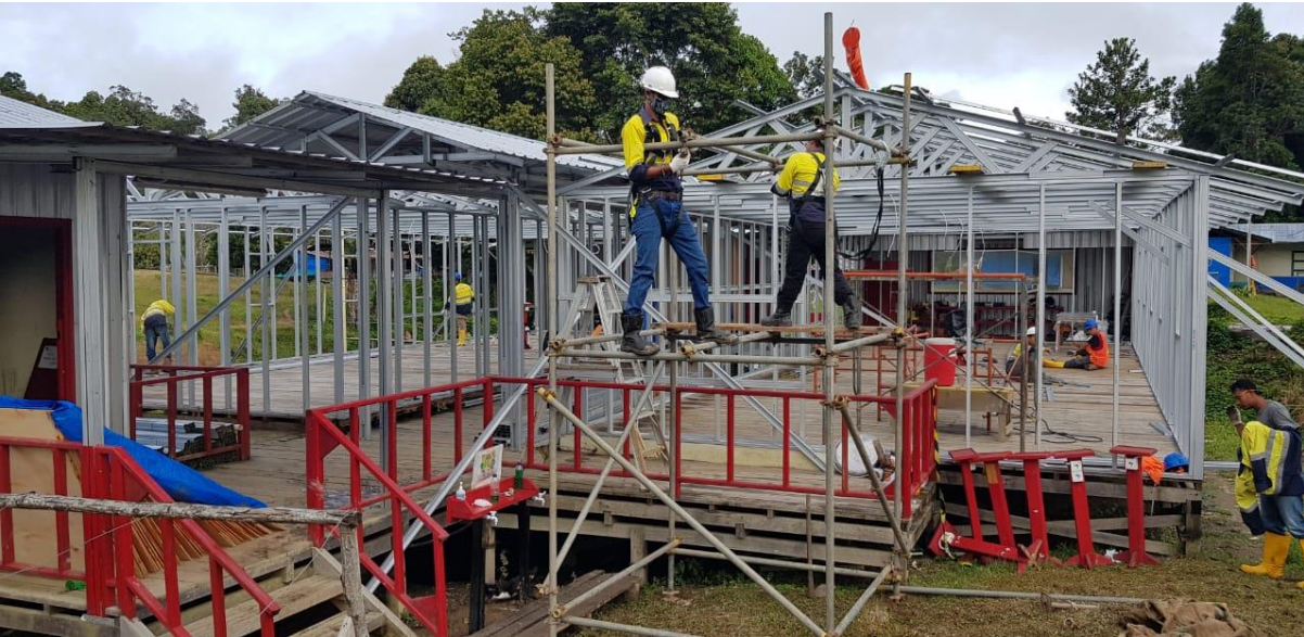
Figure 18: Upgrades to the Sihayo camp
