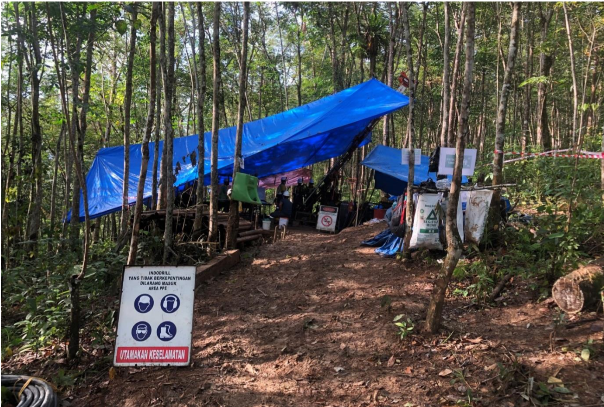
Hutabargot Julu drilling activities
