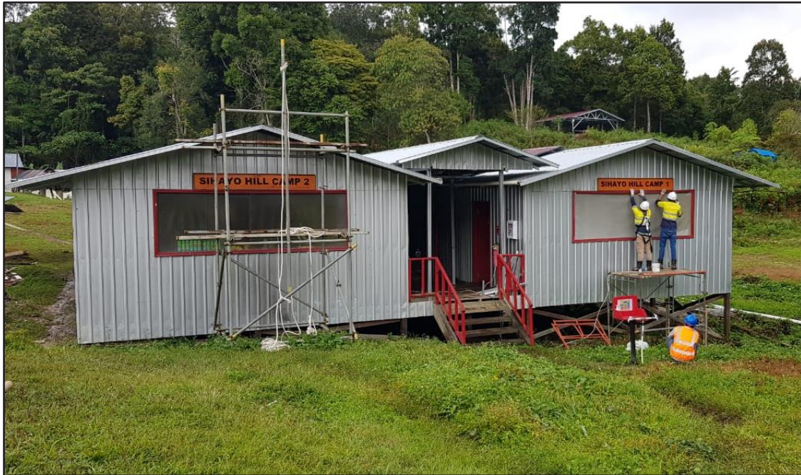
Figure 11. Refurbishment of the Sihayo Exploration Camp has been completed
