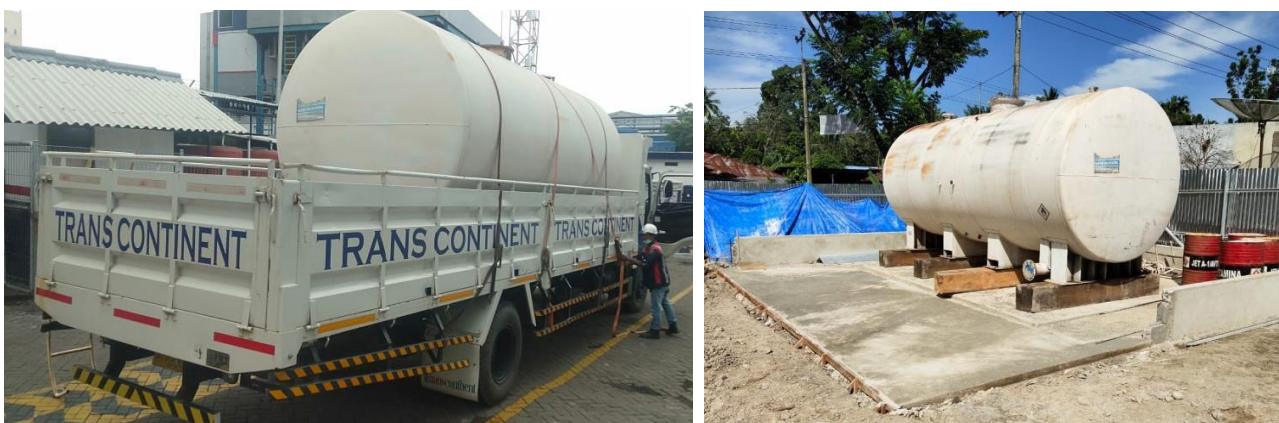
Figure 13. Delivery and installation of the 30kL fuel farm at Malintang
