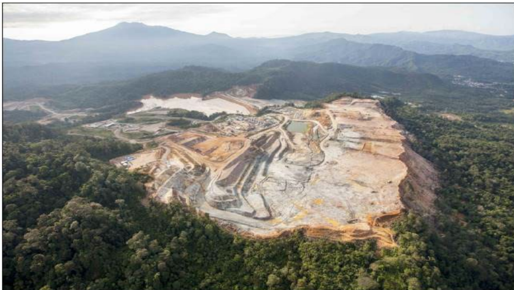
Figure 16-14. Martabe Mine Terrace Mining
