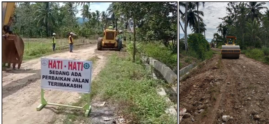
Figure 9. Sihayo Starter Project Early Works – Widening of existing access
